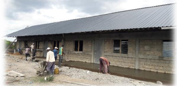
Finishing the verandah of the 3 classrooms and 2 offices
