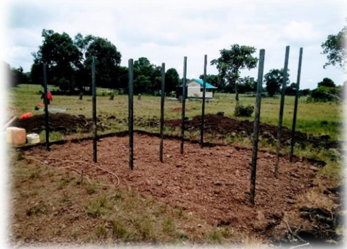
The slab is now poured and frames up
